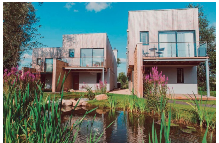
Image 6: Water features are situated alongside housing to bring nature closer to people.
