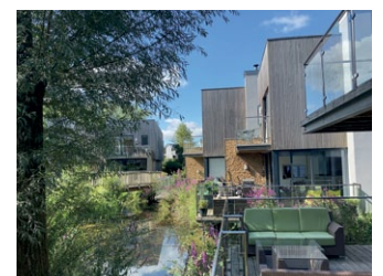
Image 4: Water is viewed as an attractive asset within the design
