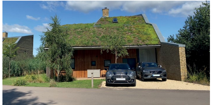
Image 12: Habitat First Group offer a range of house types to reflect the character of the estate, and enhance biodiversity measures, such as this 'Habitat House' (above) is proving to be popular and offers a green roof or wildflower turf roof
